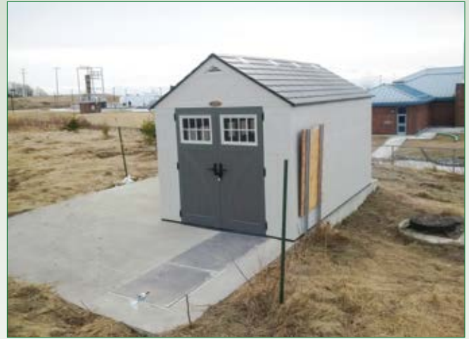
Courtice WPCP Upper Vault. 2 Odorox® units installed within off-the-shelf housing structure
