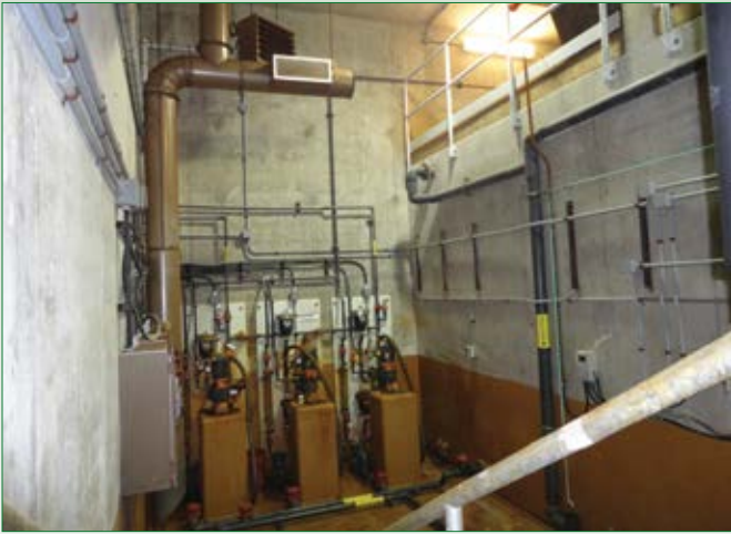
Courtice WPCP Chemical Room being treated. Odorox® Induct units servicing chemical room through existing ductwork.
