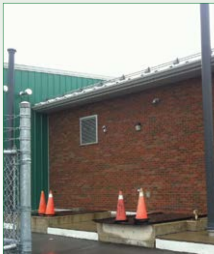
Sarnia SPS before any odour control.
