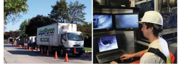
TRENCHLESS LATERAL LINING
