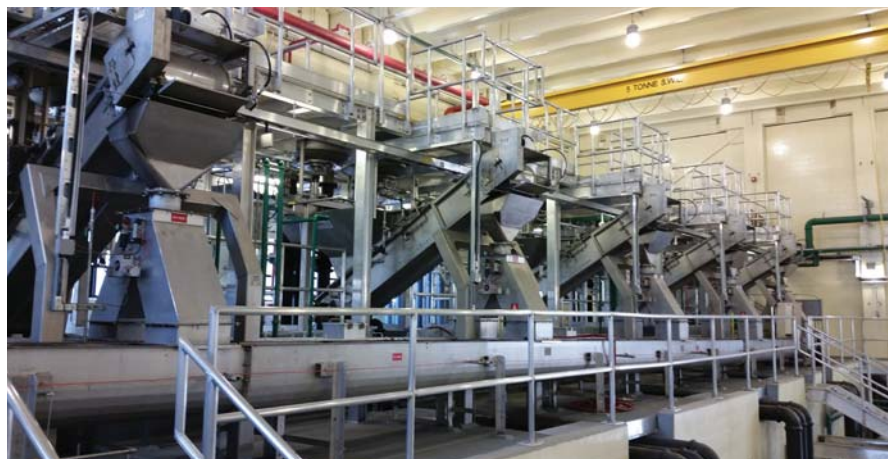
Ten Hydro SlurryCup™ Grit classifiers and five GritSnail® dewatering units treat an average flow of 418 MLD 110 MGD
