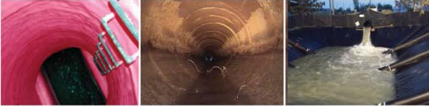
2 KM LARGE DIAMETER PIPE LINING - ENVIRONMENTALLY SENSITIVE
