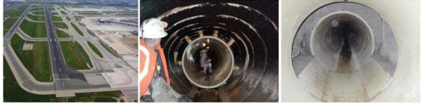
LARGE DIAMETER GRP PIPE LINING
