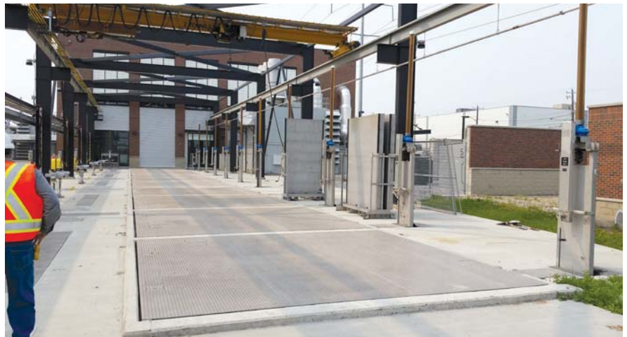
Hydro International's HeadCell® grit removal units are installed under protective covers
