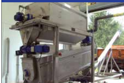
DSP Screw Press Model 3012, NY WWTP
