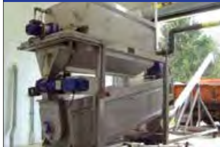
DSP Screw Press Model 3012, NY WWTP
