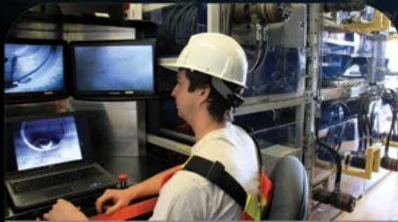
Totally Trenchless Lateral & Mainline Lining
