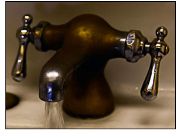
Brass Fixtures, pre- 2014 can contain up to 8% lead
